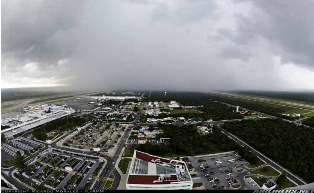
Figure 1. Heavy Rain at Cancun Airport
